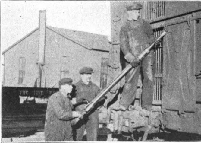
Fig. 20. Cutting Off End Door Roller Castings.
