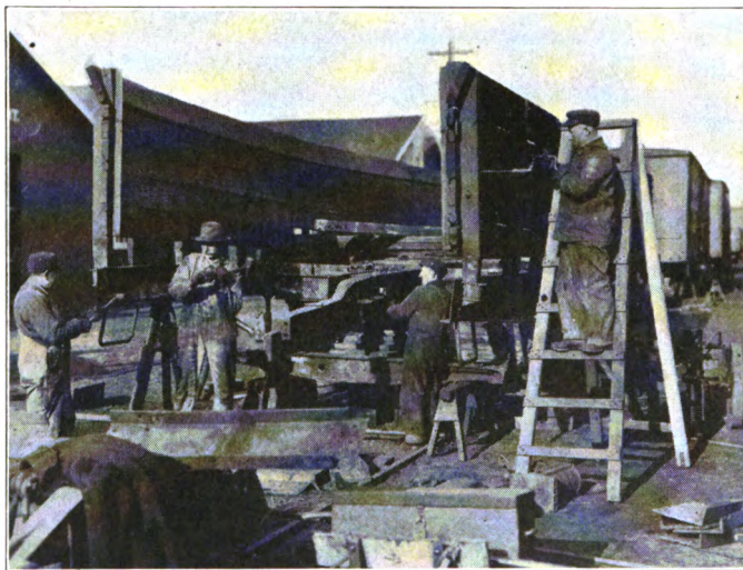
Fig. 2. Repairing a Steel Underframe Gondola Car.
