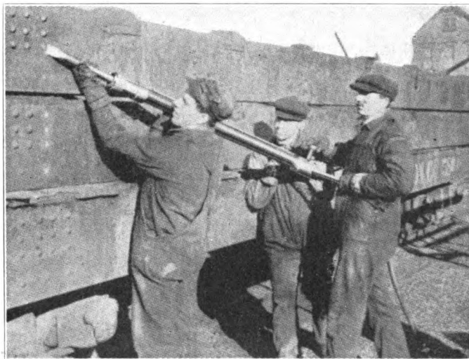
Fig. 19. Cutting Rivets from Side of Gondola Car. (Note that chisel must be held.)
