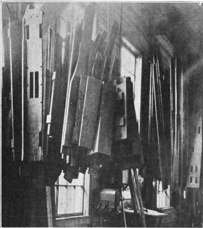
Fig. 56. Some of the Templates Made by the Layer-Out.
